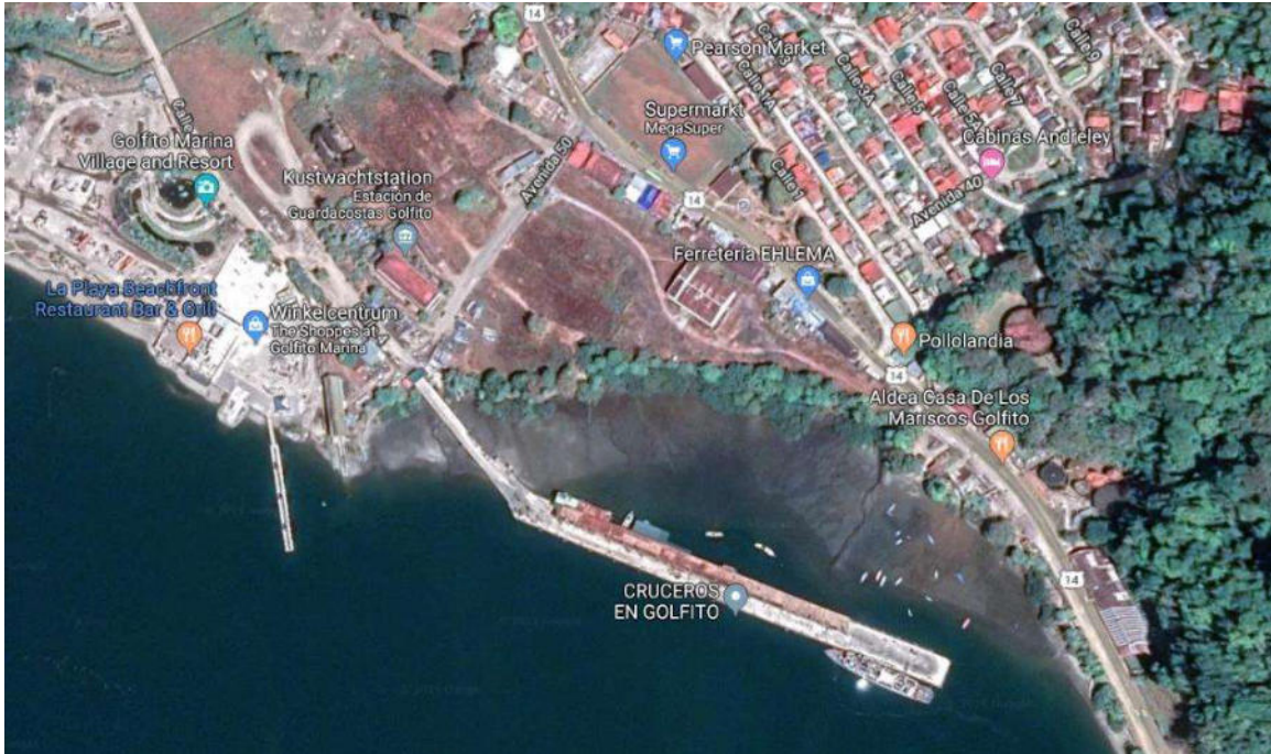
Figura 3-5 Puerto Golfito, muelle
